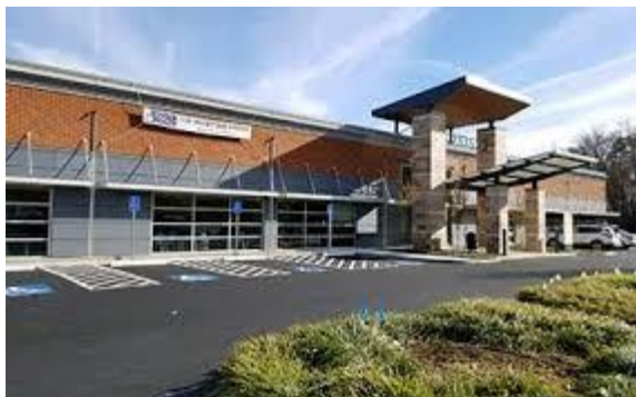
Our office Location on 29 North ( Inside UVA Primary Care Riverside Building)
